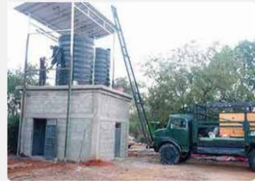
Institution Solar Water Pumping
