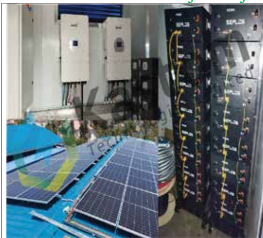
24 KWp Jinko | 24KW Jinko | 40 Kwh SEPLOS MGAS Utawala e-bike charging station
